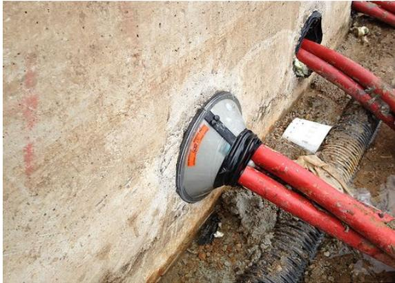
Duct sealing system type MD 2 has been developed to provide an effective and simple solution for all your Gas and Watertight duct sealing requirements. Seals internally & externally around the outside edge of the duct
