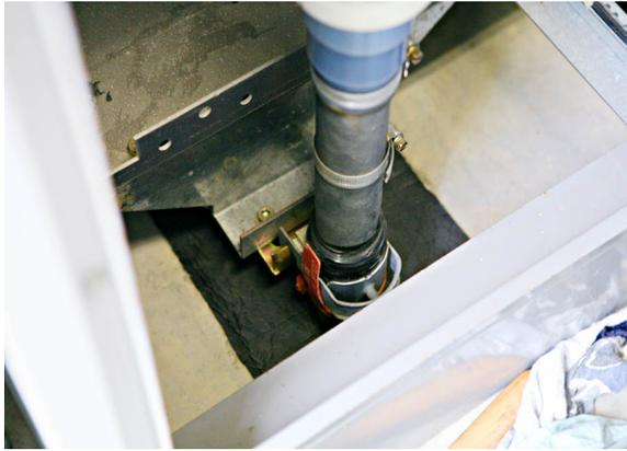
The Filoform Foam Plate is a closed cell, cross-linked polyethylene foam. The product can be easily shaped with a knife to fit into a floor or duct opening. The foam will prevent humidity to access stations. The foam can be fixed to walls and cables with use of the Filoform Hyperflash tape. Creates an airtight seal to prevent humidity problems. Easy to cut. Flame retardant.
